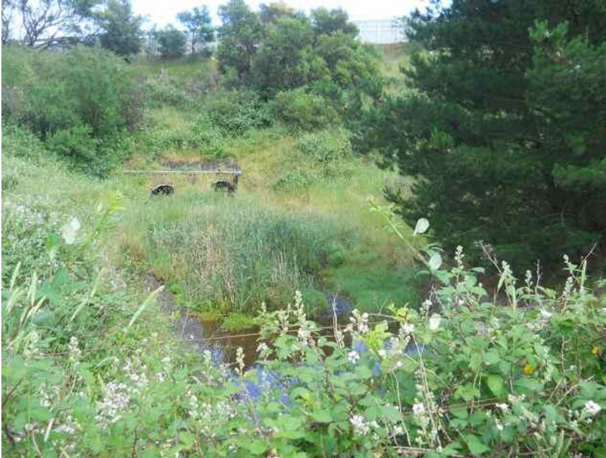
Figure 16, Tuerong Ck culvert under Mornington Peninsula Fwy. Photo taken on border between Dromana Estate and property no. 7
