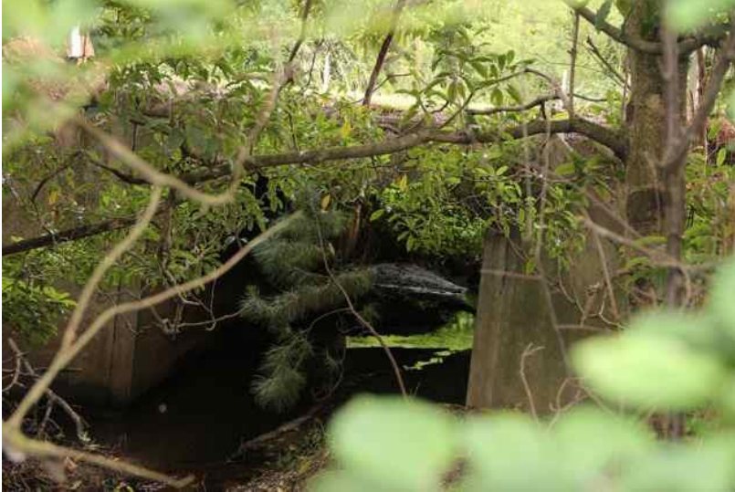
Figure 15, Devilbend Ck culvert, Old Moorooduc Rd
