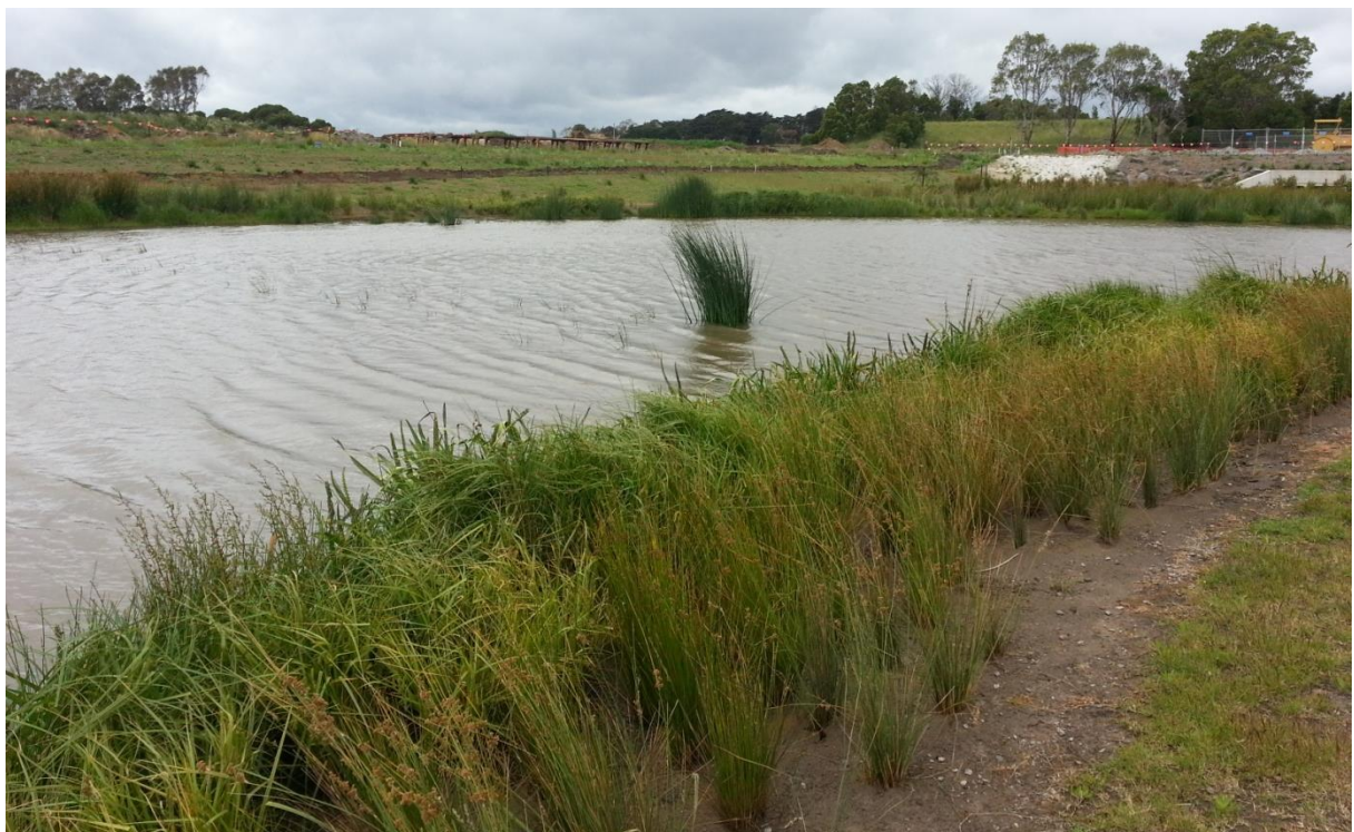
Water edges often require the highest density of plant installation. There are 6 plants per m 2 here to aid in erosion control and recreate habitat, particularly for frogs and birds. Source: Wetland Wildlife Creations Pty Ltd
